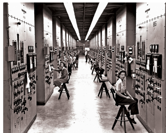
Fig.3. Young women operating calutron, the heart of the uranium electromagnetic separation process, at Y-12 plant in Oak Ridge, Tennessee. (in a US government photo by Ed Westcott). 19,20
